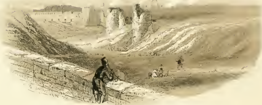
Inner Breach looking south
